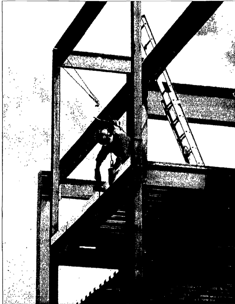
A Weyerhaeuser construction worker welds together the skeletal structure of the latest Whitworth building project.
