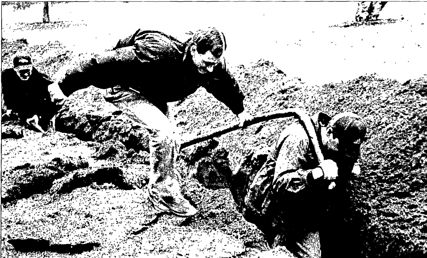
Whitworth students juniors Patrick Plumb and Tom Yochum help Joe Graham lay fiberoptic lines as part of the Dixon Hall renovation.
