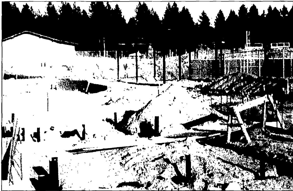
Construction is underway on the new athletic fields on the west end of the Whitworth campus.
