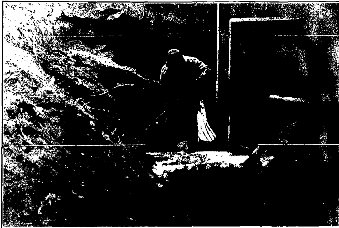
A library construction worker digs in the area of the foundation of the new library wing. Construction is a week behind schedule, but Library Director Hans Bynagle said there is a good chance the completion will end up ahead of schedule.
