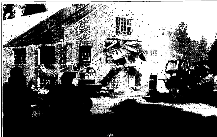
Keith Sullivan and Ed Eccles of the Physical Plant watch as the library gets demolished last fall. The new wing is almost finished.
