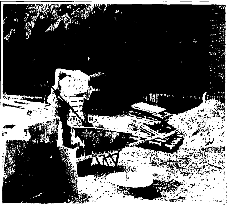
A construction worker prepares Mac Hall for its residents' Sept. 5 arrival.
