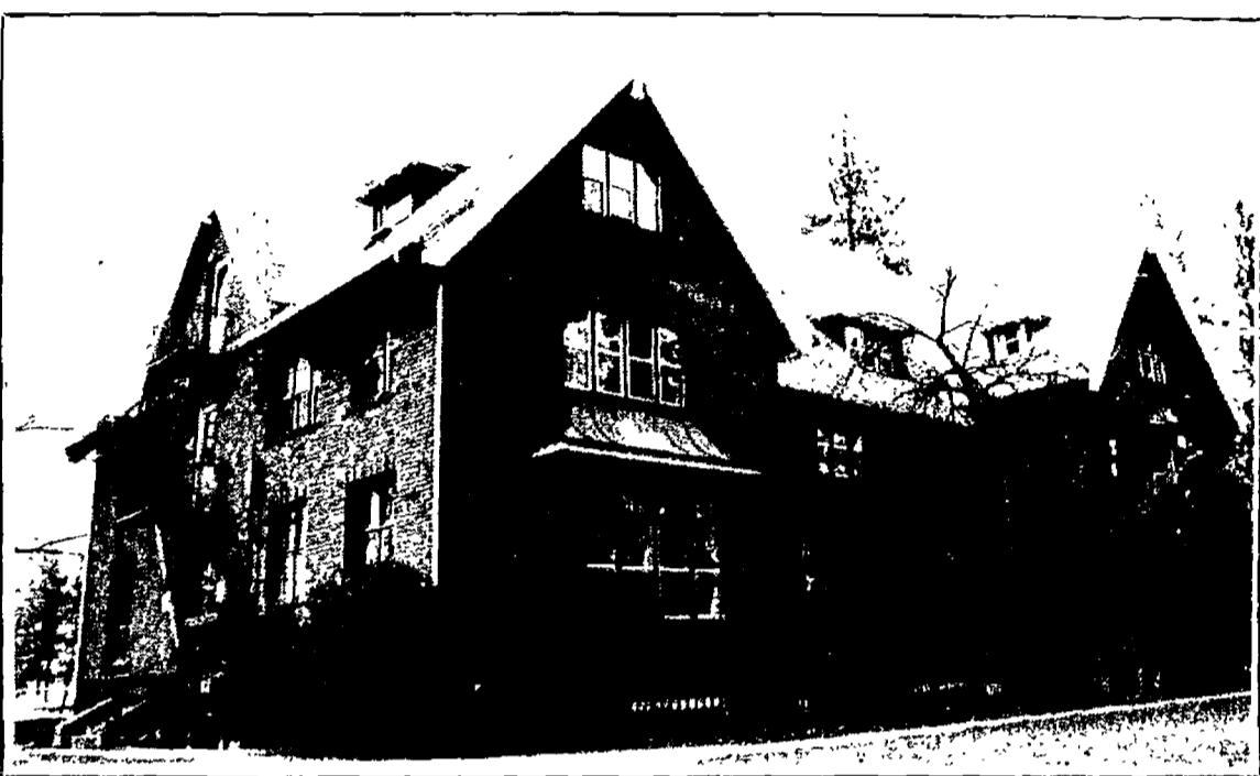
McMillan Hall undergoes renovations beginning May 19.
