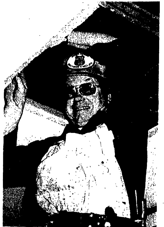
A workman renovates Dixon Hall.
