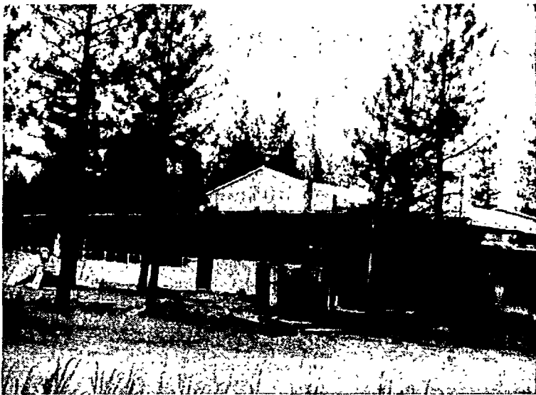
'Into Reality' comes the long awaited HUB. Pictured above is a portion of the new building that has been under construction since last fall. It will be ready for use at the beginning of the fall semester.
