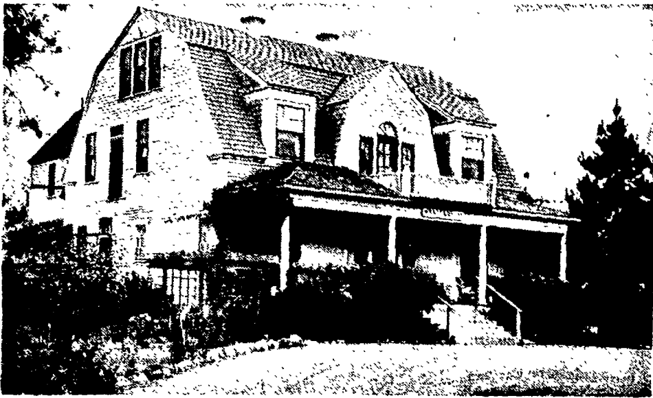
Whitworth hall has been leased by the college as a men's dormitory. At present 32 men of the college claim this as their home. It is filled to capacity. The home economics laboratory is in the basement of the building.
