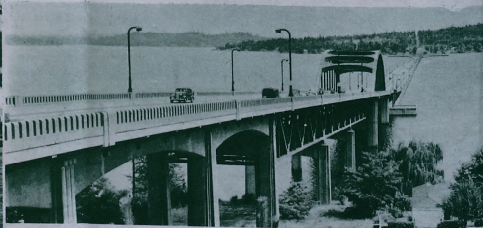
Famous floating bridge on Lake Washington connecting Mercer Island with the mainland. A movable span permits navigation to pass from one part of the lake to another.
