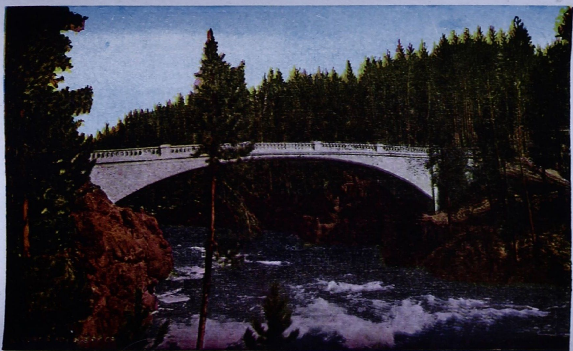
4507. Chittenden Bridge, Yellowstone National Park
