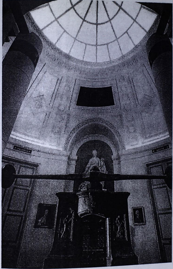
Illustration 46. Apse of the main foundry room, containing the statue of Fortune, in the foreground the screw press of Louis XIV, dating to 1699. From Rachline, 30.
