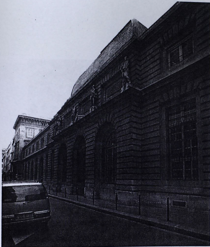
Illustration 31. Central bay, side façade, looking south. Photo courtesy of Leland M. Roth, 2003.
