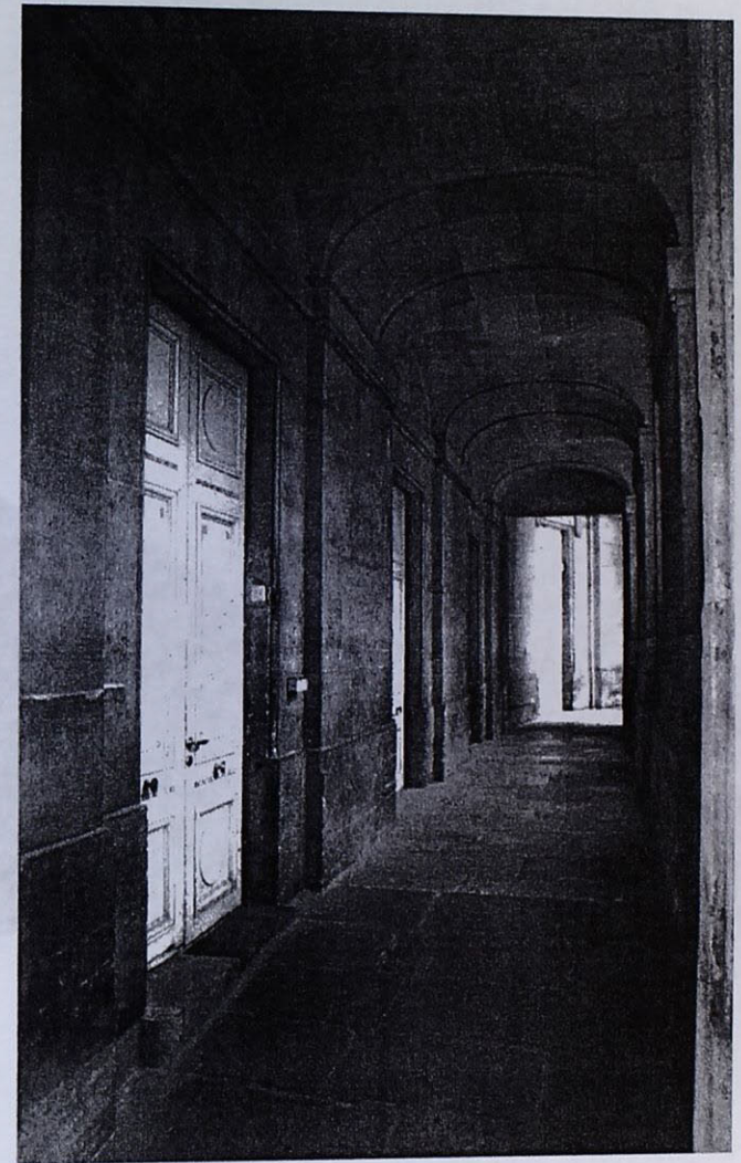
Illustration 55. Main court curved passage, looking south. Photo courtesy of Leland M. Roth, 2003.
