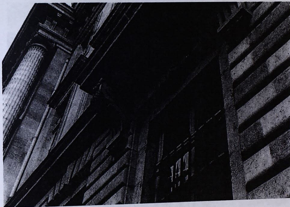
Illustration 58. J.-D. Antoine, window-bracket detail, main façade, Hôtel de la Monnaie, Paris, 1765-1775. Author's photograph.
