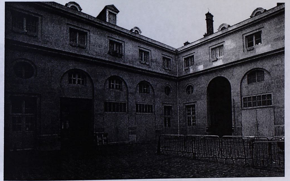
Illustration 51. Western side court, looking southwest. Modifications have been made to some of the entry doors. Photo courtesy of Leland M. Roth, 2003.
