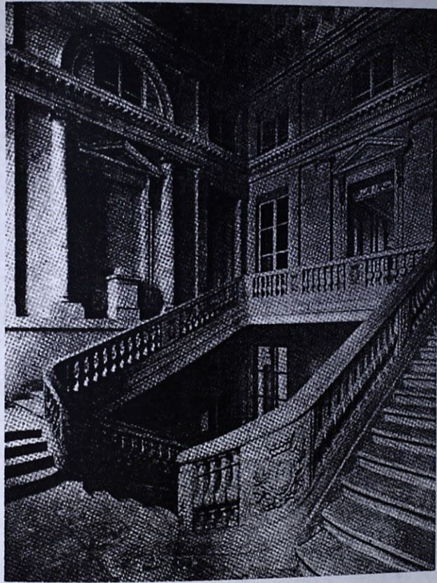
Illustration 41. C.-N. Ledoux, grand stair, Château de Bénouville, Normandy, 1770-1777. From Middleton and Watkin, 150. The authors compare this stair to Antoine's, page 142.
